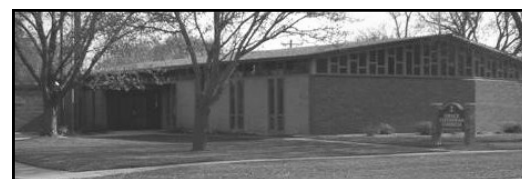
Grace Lutheran Church 380 N. Rerick Avenue, Primghar (712) 957-4795
